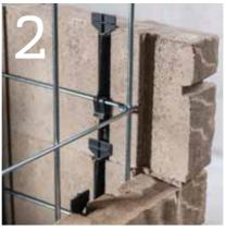
Use connector to attach Lafitt Tandem™ Ashlar Unit to grid
